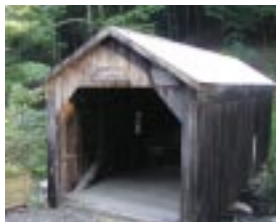
Copeland Covered Bridge, Edinburg
